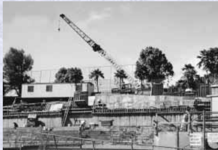
Kapālama's Ke'elikōlani Swimming Pool renovation
