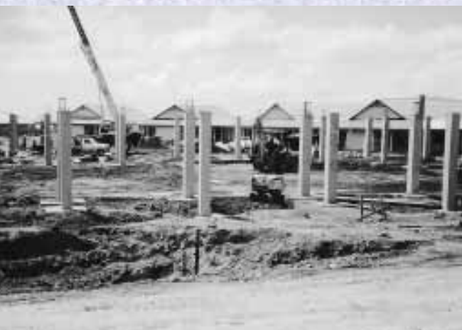
Maui Campus' cafetorium under construction
