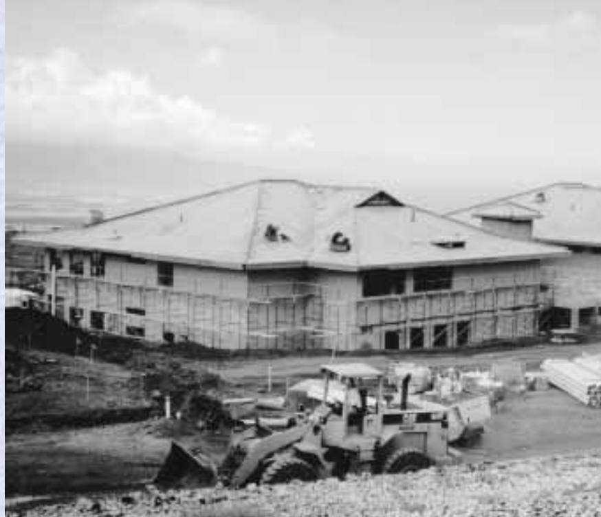
The Administration/Library Building on KSBE's new Maui Campus.
