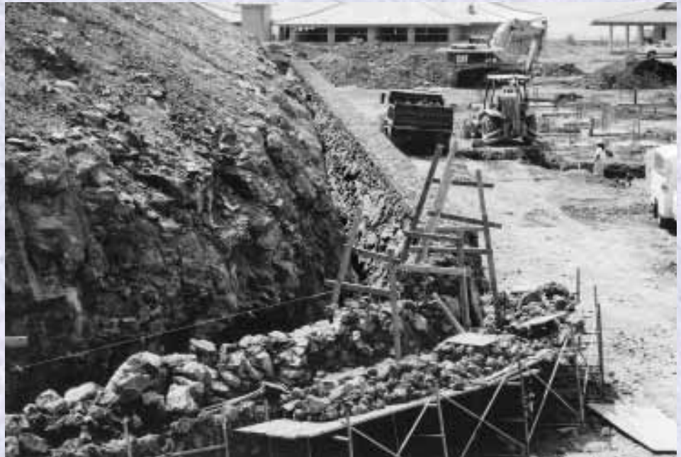
A view of the Maui Campus Administration Building/Library over lava rock wall construction.
