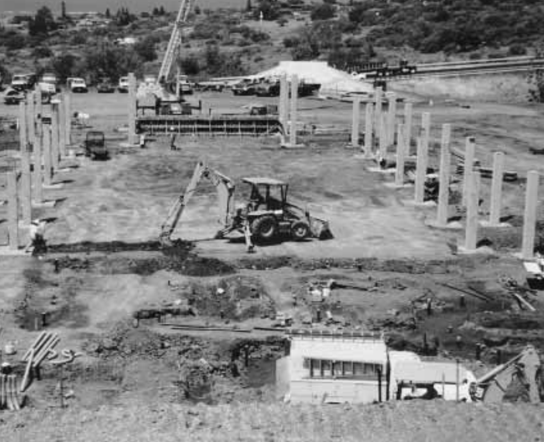
Maui Campus' cafetorium under construction.
