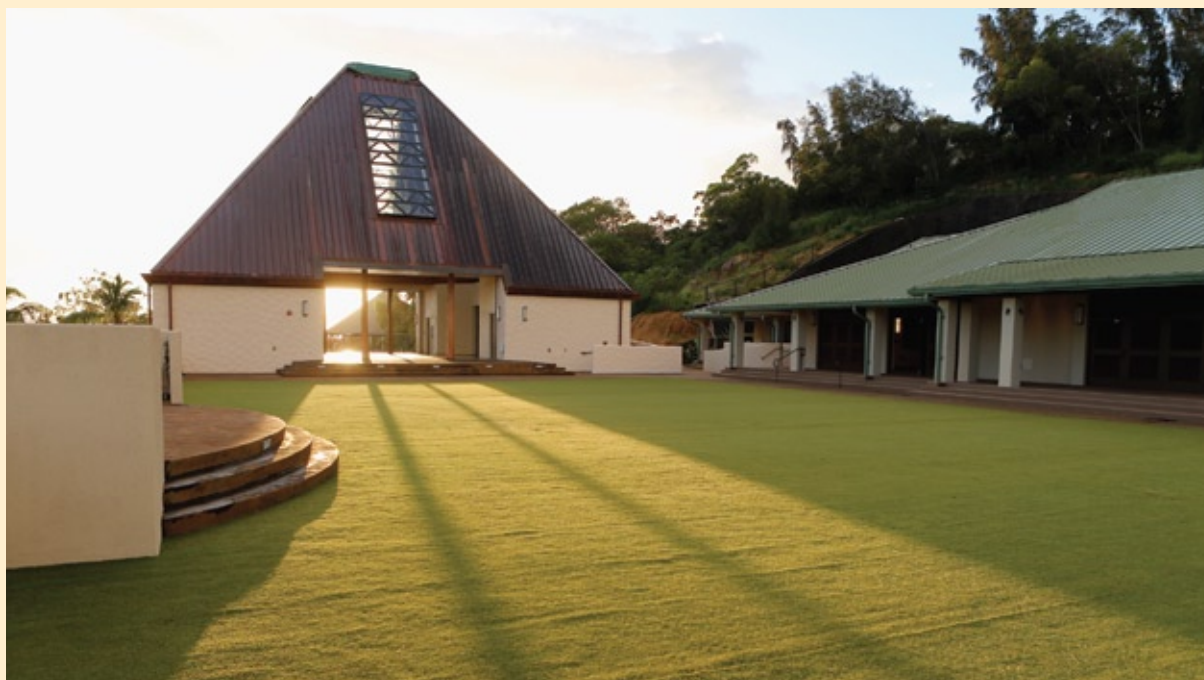
Major construction on the Ka'iwakiloumoku Hawaiian Cultural Center, located on the Kamehameha Schools Kapālama campus, was completed in fiscal year 2012. The center is part of the school's $118 million Ke Kupu Mālamalama campus renovation project.
