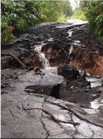
Water erosion on Mauna Loa Road in Aloha Estates.
